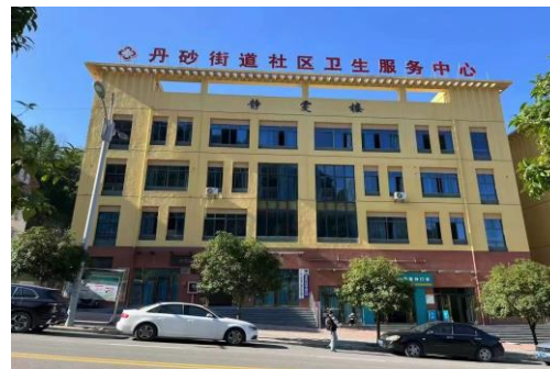
Construction of medical centre
