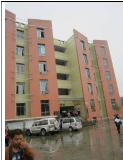
Sponsor school Building
